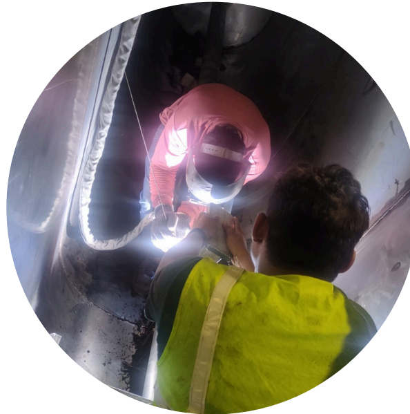
OWC MACHINE MODIFICATION
